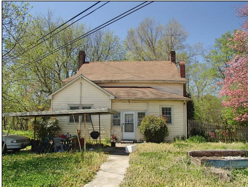
12: Caldcleugh House, east elevation and carport
