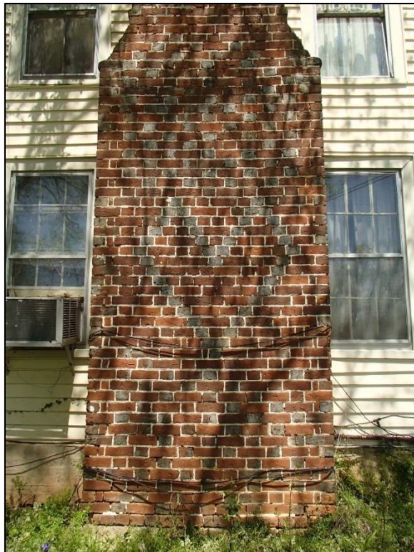
9: Caldcleugh House, south elevation chimney detail
