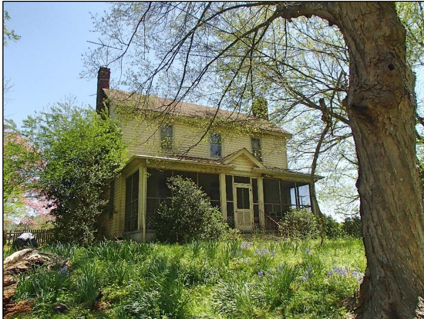
4: Caldcleugh House, west elevation
