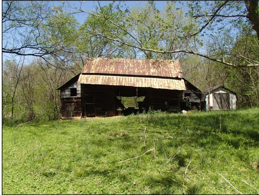
13: Caldcleugh House, barn, south elevation
