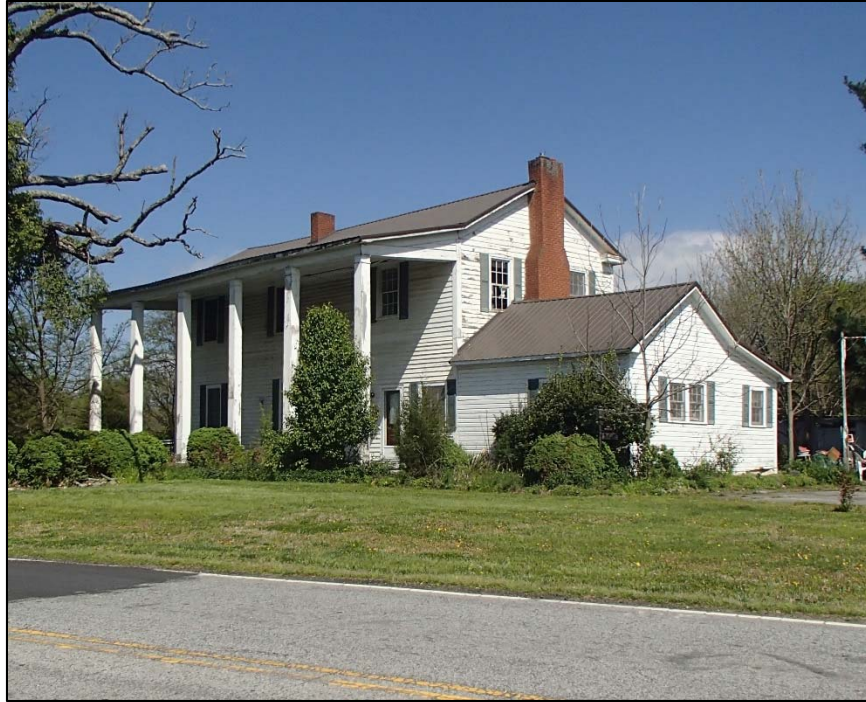
25: Unsurveyed House, corner of Junior Home Order Road and Old Linwood Road
