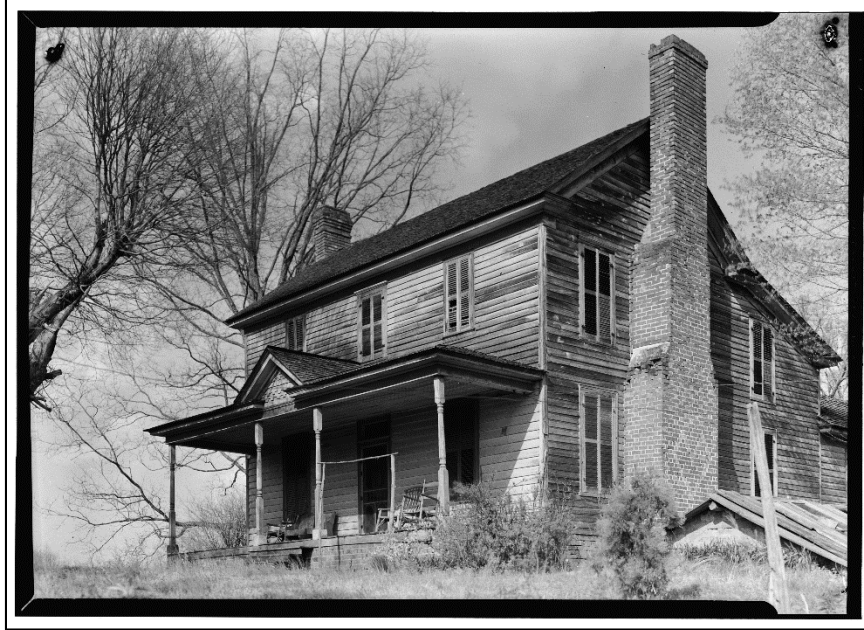
3: Caldcleugh House, Historic American Buildings Survey Photograph by Thomas Waterman, 1940
