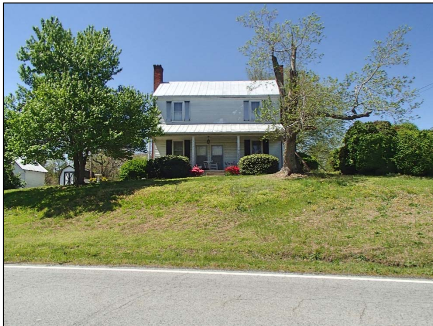
20: Saintsing House, Old Greensboro Road
