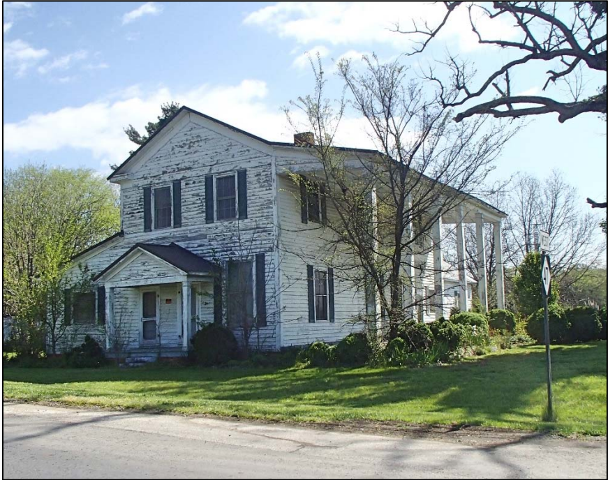
24: Unsurveyed House, corner of Junior Home Order Road and Old Linwood Road
