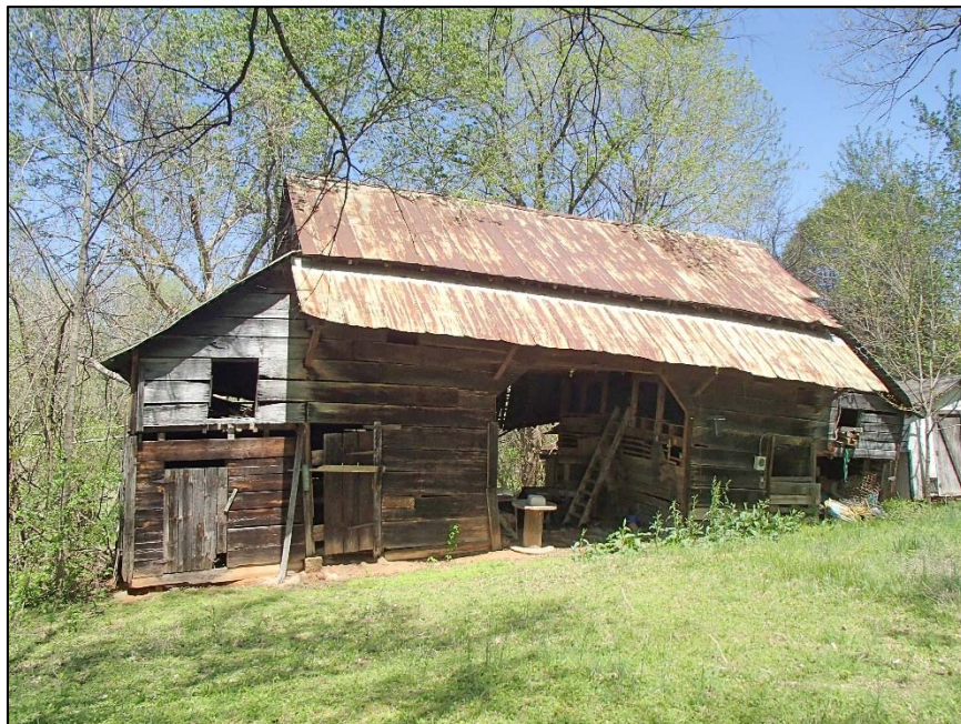
14: Caldcleugh House, barn, south elevation
