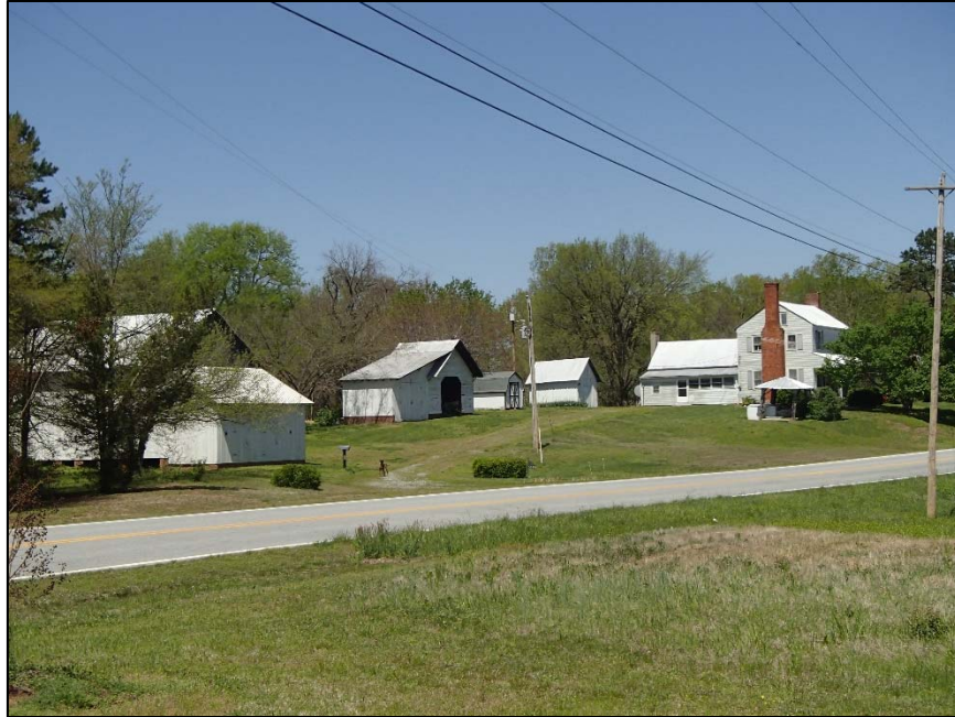
19: Saintsing House, Old Greensboro Road
