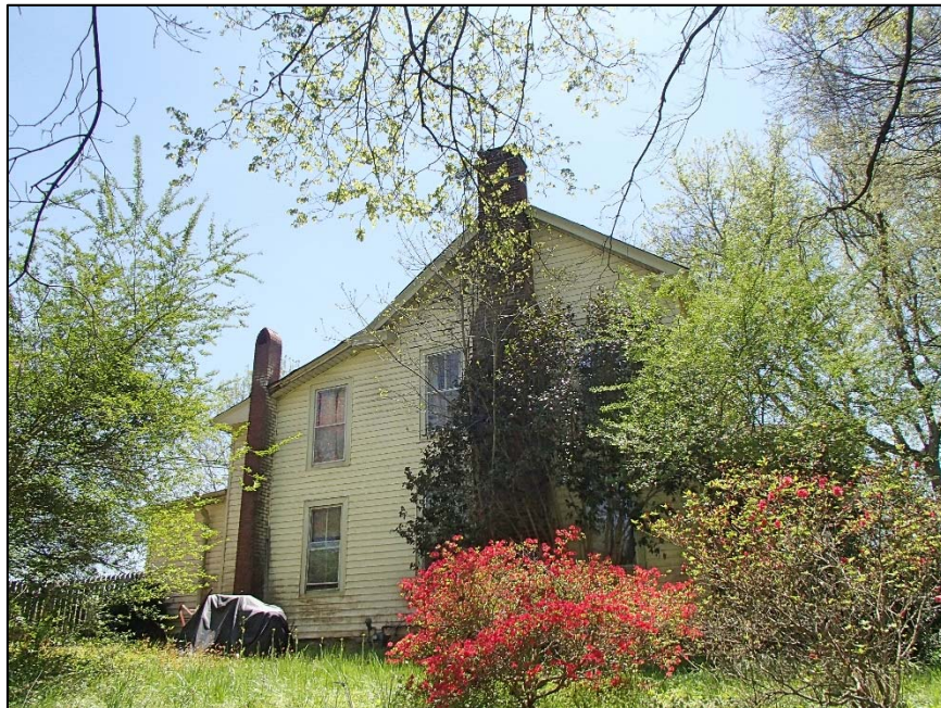
11: Caldcleugh House, north elevation
