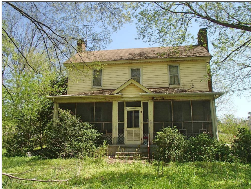
2: Caldcleugh House, west elevation
