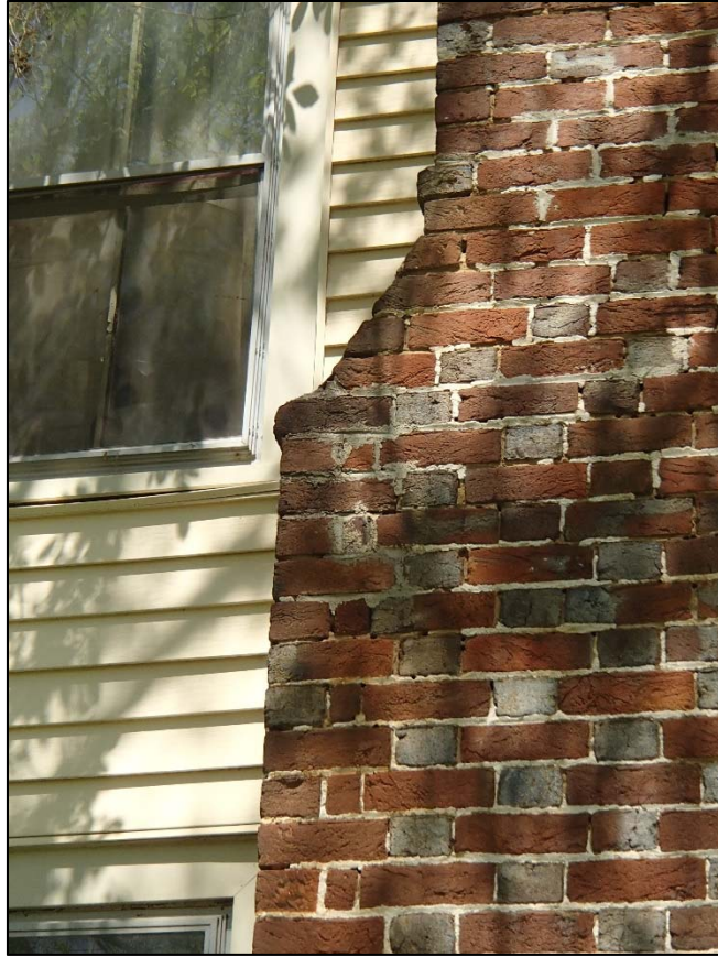
10: Caldcleugh House, south elevation chimney detail
